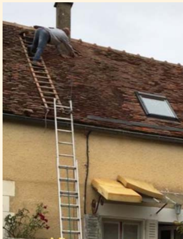
Yonita's cottage roof
